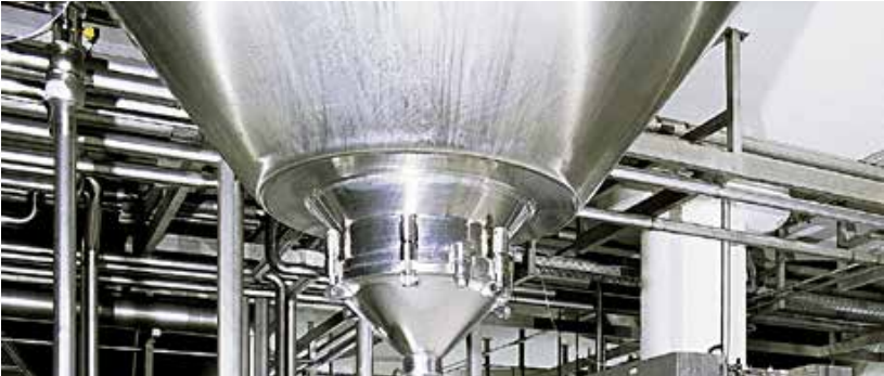
Tank and plant construction
