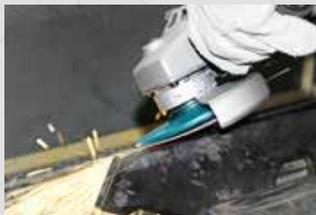
Levelling of welded seams
