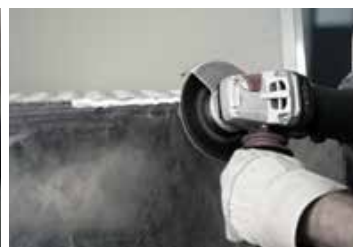
Removing welded seams
