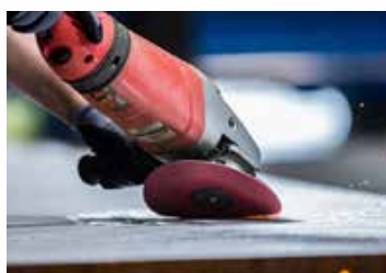
Removal of imperfections
