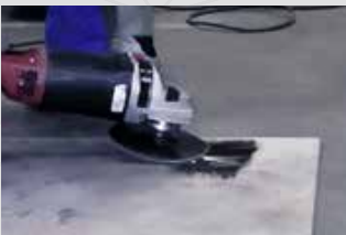
Removal of imperfections
