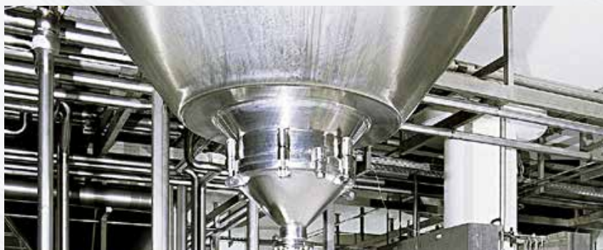
Tank and plant construction
