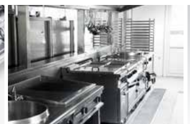
Large catering facilities
