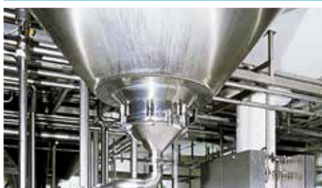
Plant and tank construction
