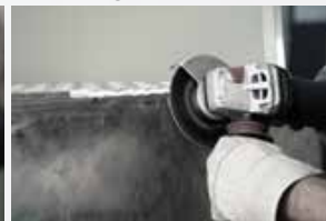
Removing welded seams
