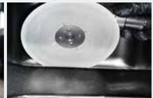
Preparing welded seams
